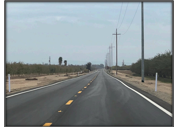
Avenue 26/Road 29 Rehabilitation
