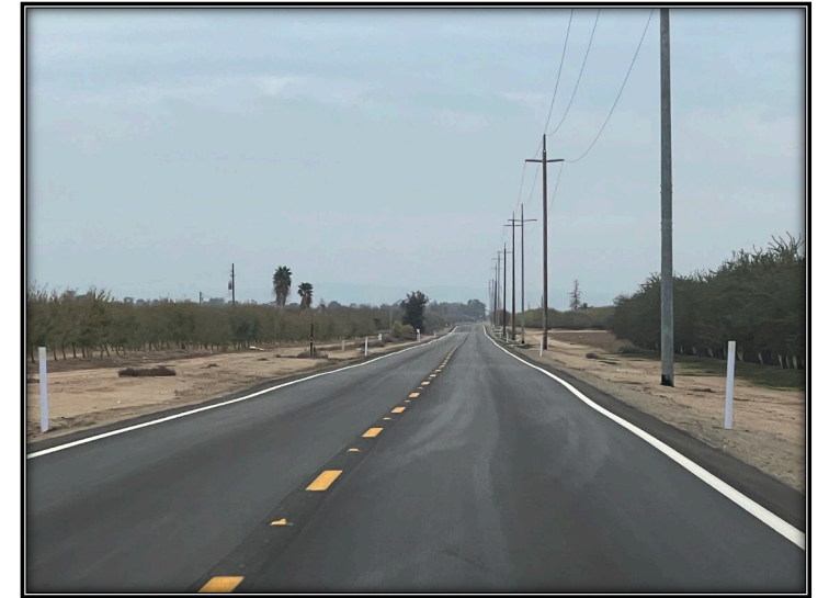
Avenue 26/Road 29 Rehabilitation
